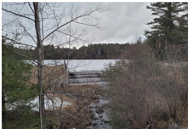
Howell's Pond Dam
